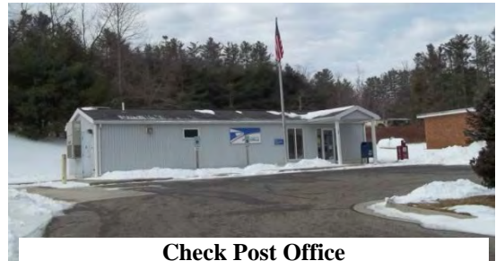
Check Post Office
