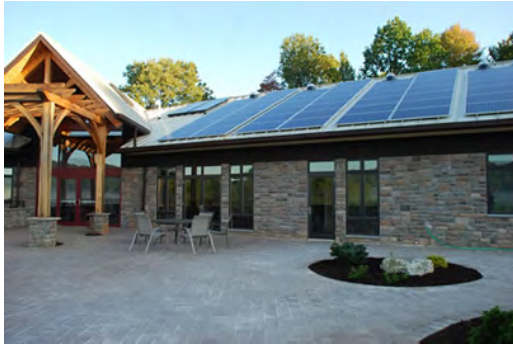
Wall Residences Office Building with solar panels, geothermal wells and grey water system
